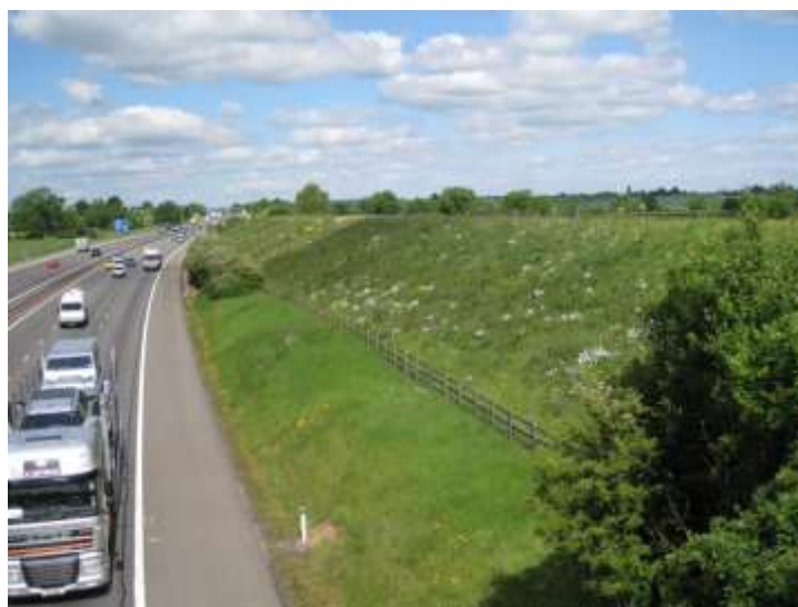
Earth bund beside the M40
